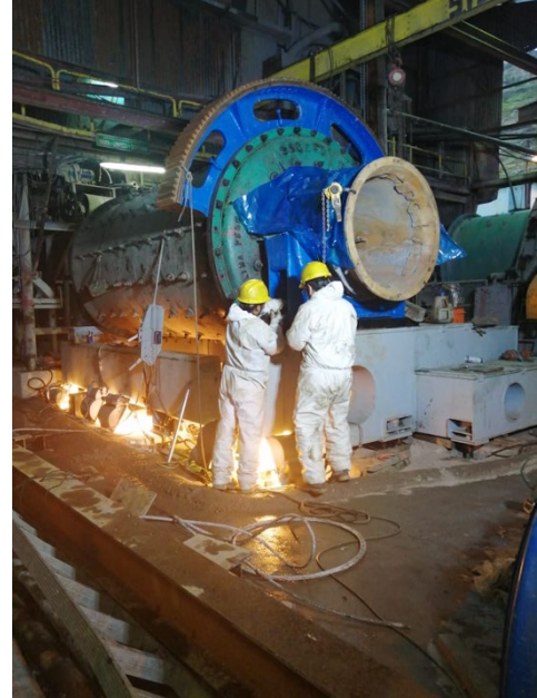
Figure 1: New mill at Nueva Recuperada Plant
